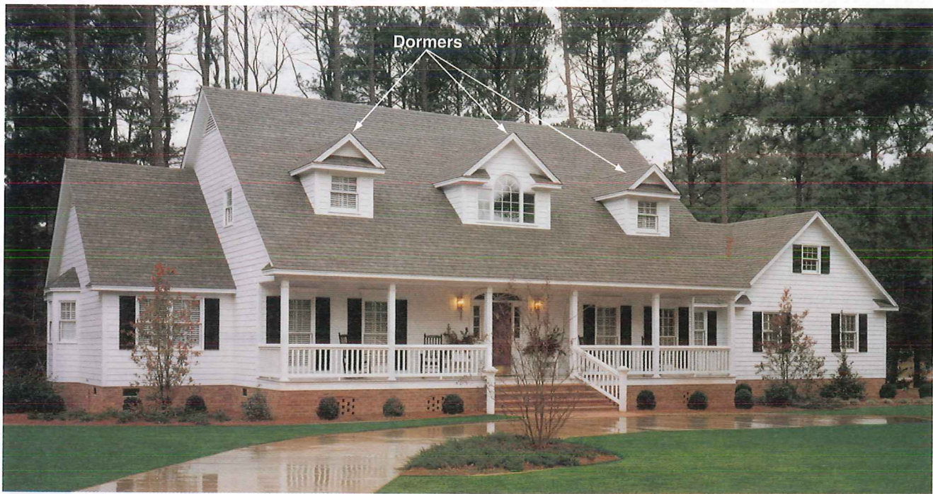
Figure 2-13. Three dormers on this attractive one-and-one-half-story house provide natural light and ventilation to the finished attic area. (Photo Courtesy of James Hardie® Siding Products)
