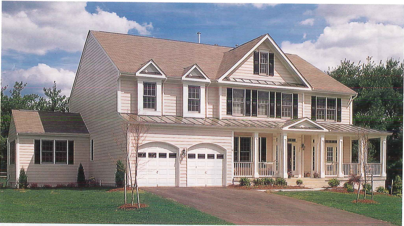
Figure 2-18. The basic two-story house takes on a contemporary appearance with an overhanging porch roof, dormers, and a small room addition. (Photo Courtesy of James Hardie® Siding Products)
