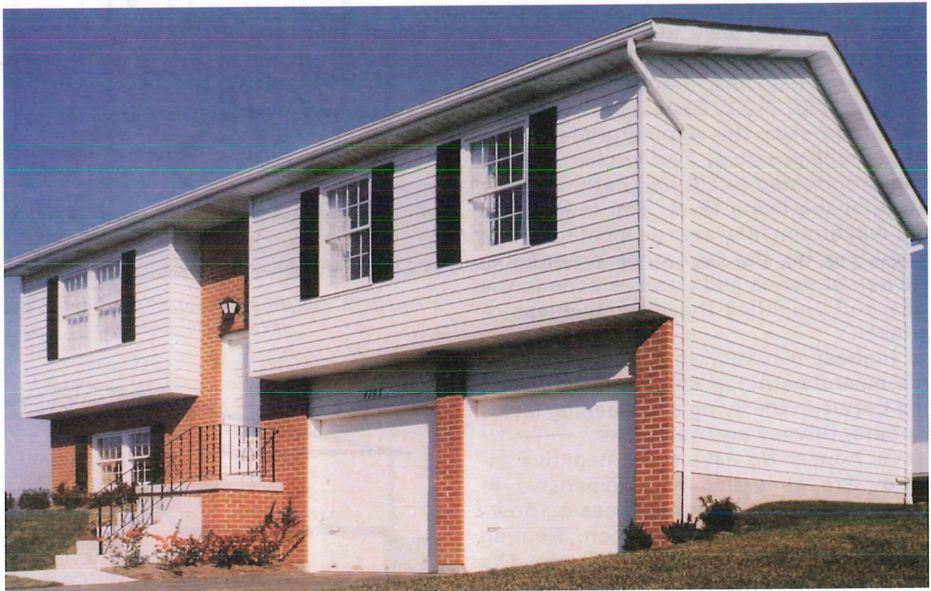
Figure 2-25. This simple design has a split entry to take advantage of a raised basement to add height and better lighting. (Aside)
