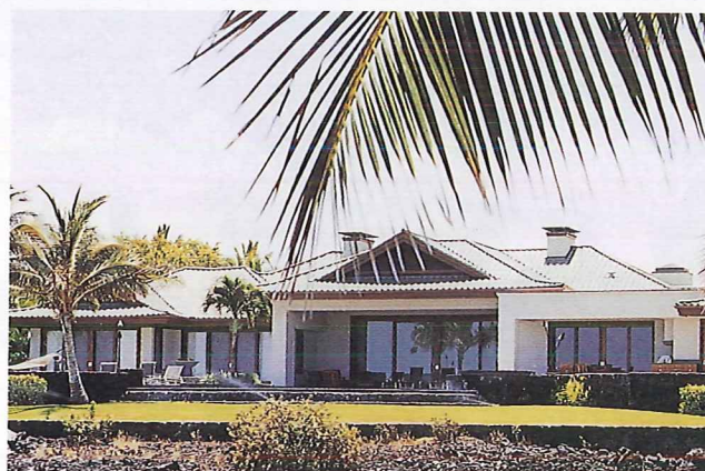
Figure 2-10. This spacious ranch house has extensive roof and wall areas that may produce maintenance problems.
