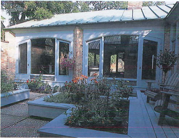
Figure 2-2. The quality of this outdoor space greatly enhances the living area of the home.
