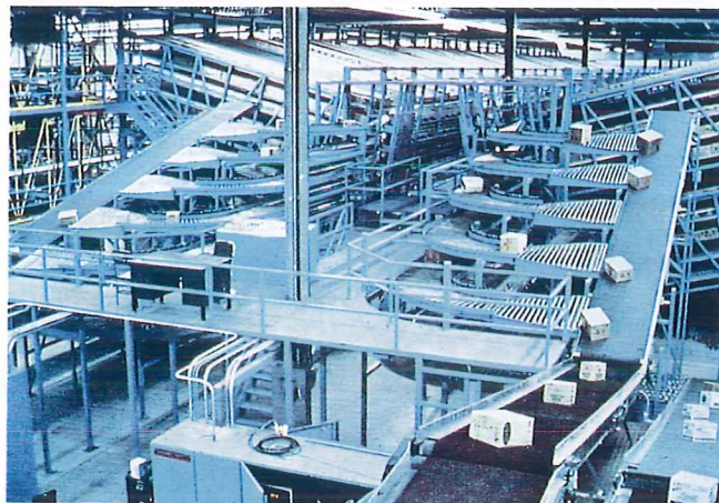
Figure 1-19. Engineers deal with systems and products that might be very complex. A material handling system used in a large distribution warehouse might involve a very complex conveyor arrangement. An engineer is needed to design a solution to this type of problem. (SI Handling Systems, Inc.)
