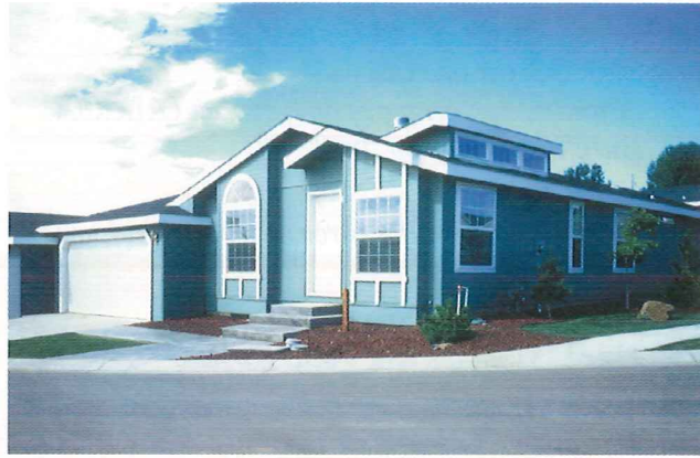
Figure 15-58. The clerestory windows shown here are a series of standard windows. (Manufactured Housing Institute)
