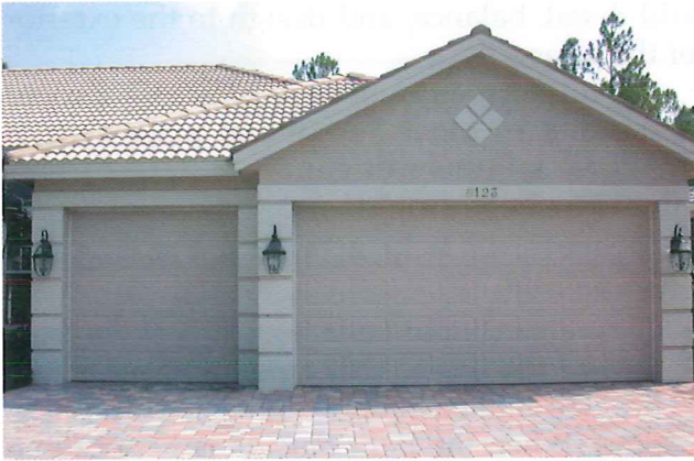
Figure 15-18. This overhead sectional garage door is made of steel.
