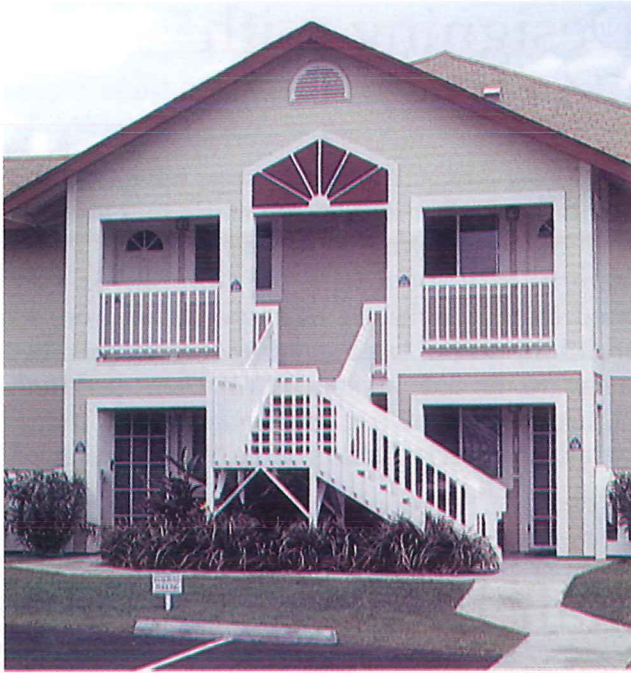
Figure 16-15. These exterior stairs are constructed at the proper angle to afford safe travel to the upper level of the condo.
