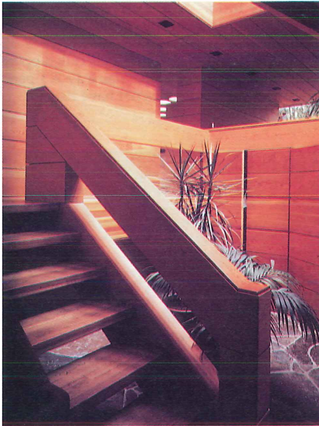
Figure 16-16. This is an open riser stairway. Notice the large treads and lack of risers. (Western Wood Products Association)
