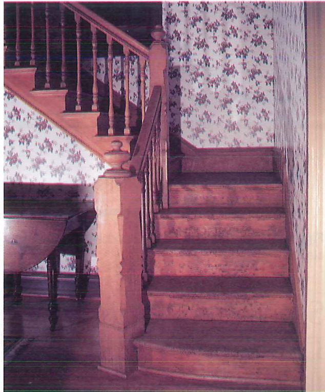
Figure 16-18. These stairs in an older home violate Rule 1 of good stair design because they slope at close to 45^\circ , rather than the appropriate 30^\circ to 35^\circ . (Brad L. Kicklighter)
