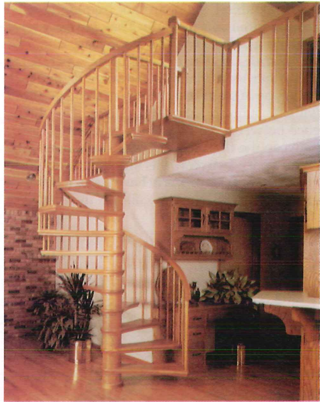
Figure 16-7. A—Spiral stairs. B— These decorative spiral stairs are made from prefabricated parts. (Arcways, Incorporated)
