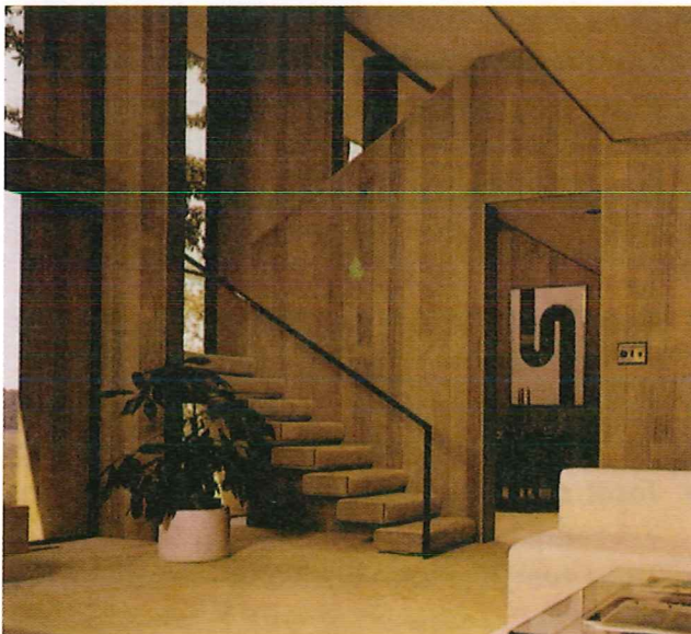
Figure 16-5. A—U stairs. B—These stairs are narrow U stairs. Notice the lack of a well hole. (California Redwood Association)
