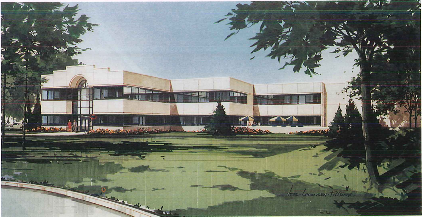
Figure 23-1. Structural drafters prepare drawings used in the construction of buildings. Precast concrete panel units were used to construct this building.
