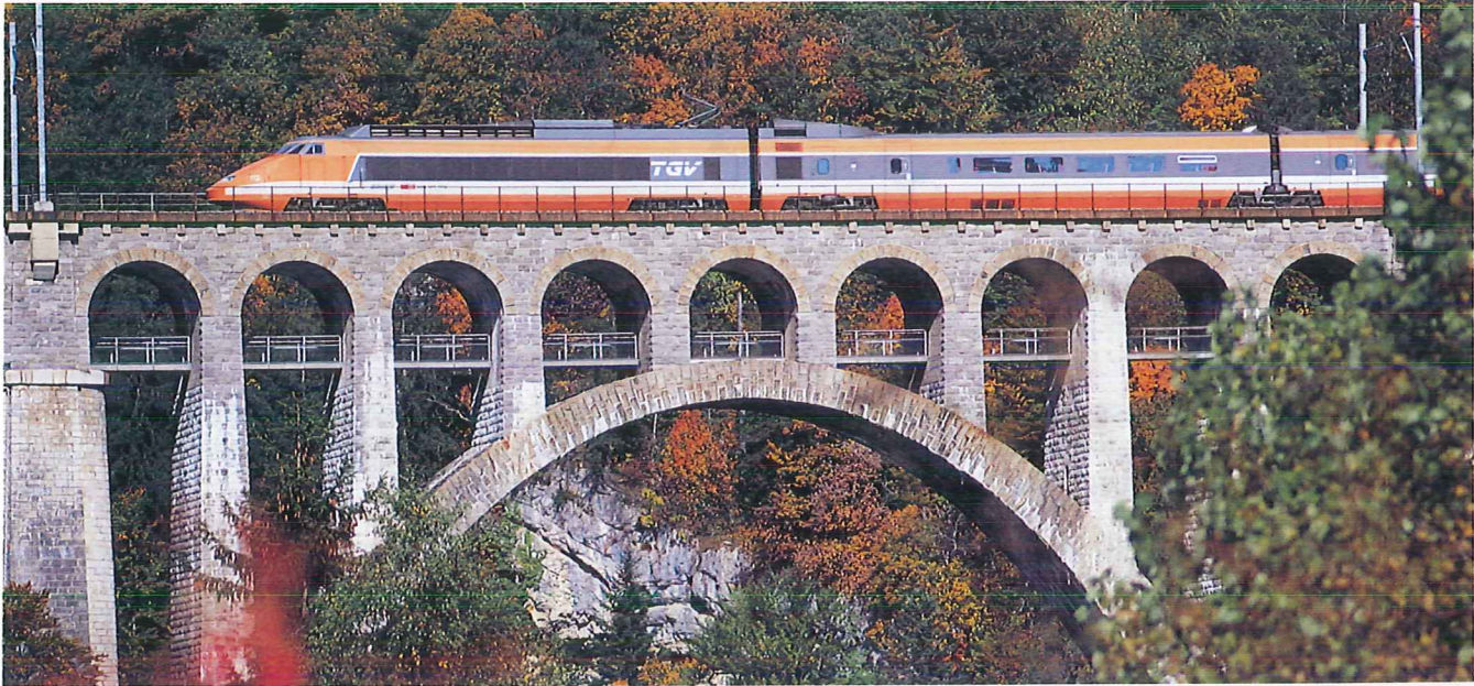
Figure 7-12. Parabolic curves are commonly used in the design and construction of bridges.
