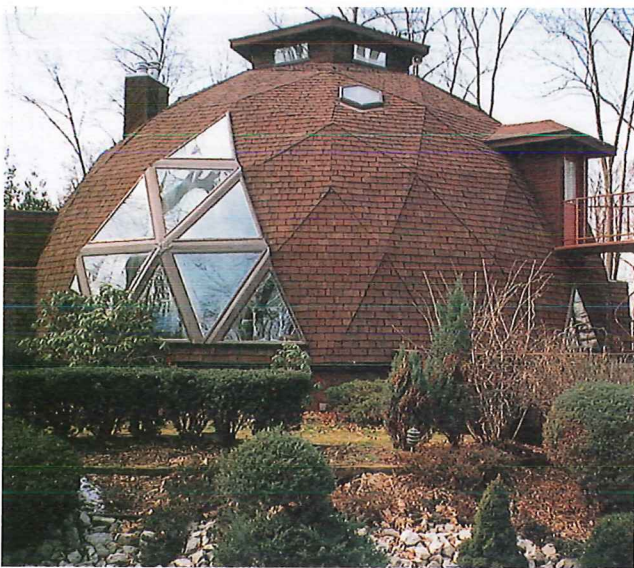
Figure 1-35. This dome home is constructed from manufactured triangular sections assembled on-site to produce the roof and walls of the structure. (Linda Lindeman)
