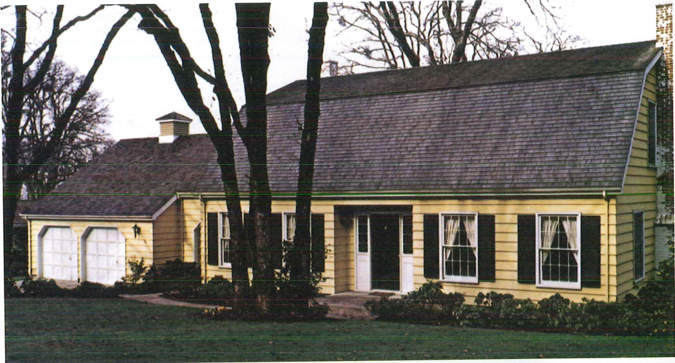
Figure 1-6. The typical New England Gambrel style is adapted to this contemporary house.
