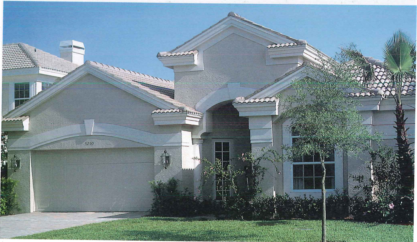
Figure 1-22. This thoroughly modern ranch home exhibits architectural detail designed to set it apart from traditional ranch homes. (Arthur Rutenberg Homes, Inc.)
