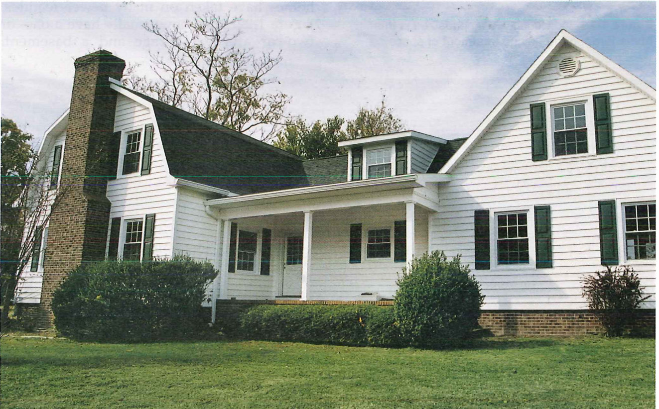
Figure 1-18. Homes can be designed to require minimal maintenance. Materials such as vinyl or solid aluminum siding, gutters, downspouts, ornamental shutters, fascia, and soffits are attractive and easy to clean and maintain. (Norandex/Reynolds Building Products)
