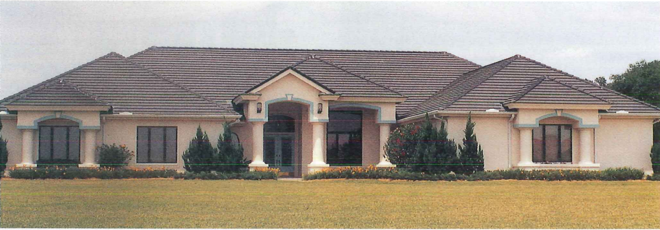
Figure 1-23. This home contains the basic elements of the ranch style yet incorporates many contemporary architecture details.
