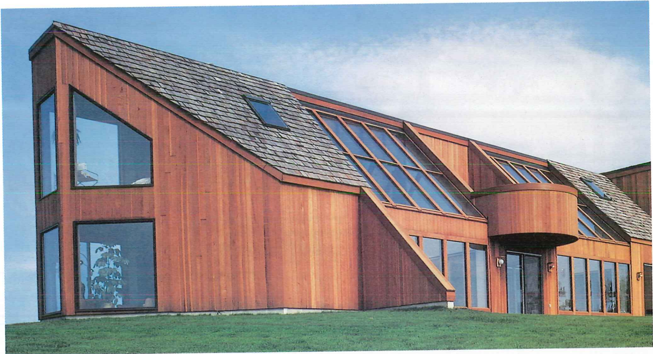
Figure 1-19. Large areas of glass are used extensively in this contemporary home. (California Redwood Association)
