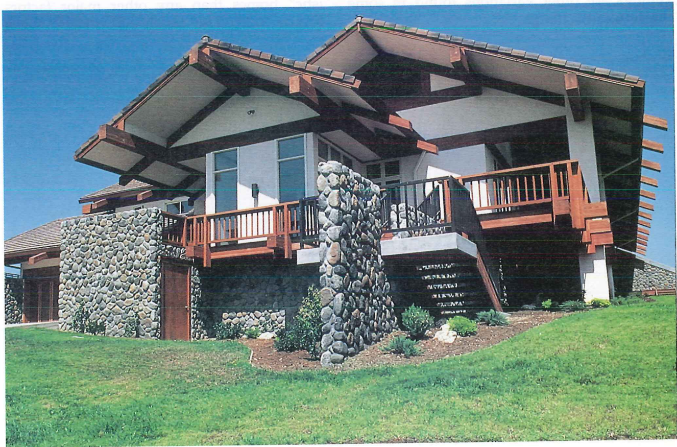
Figure 1-20. Visible roof supports are part of a dominant design element in this home. (Cultured Stone by Stucco Products, Inc.)
