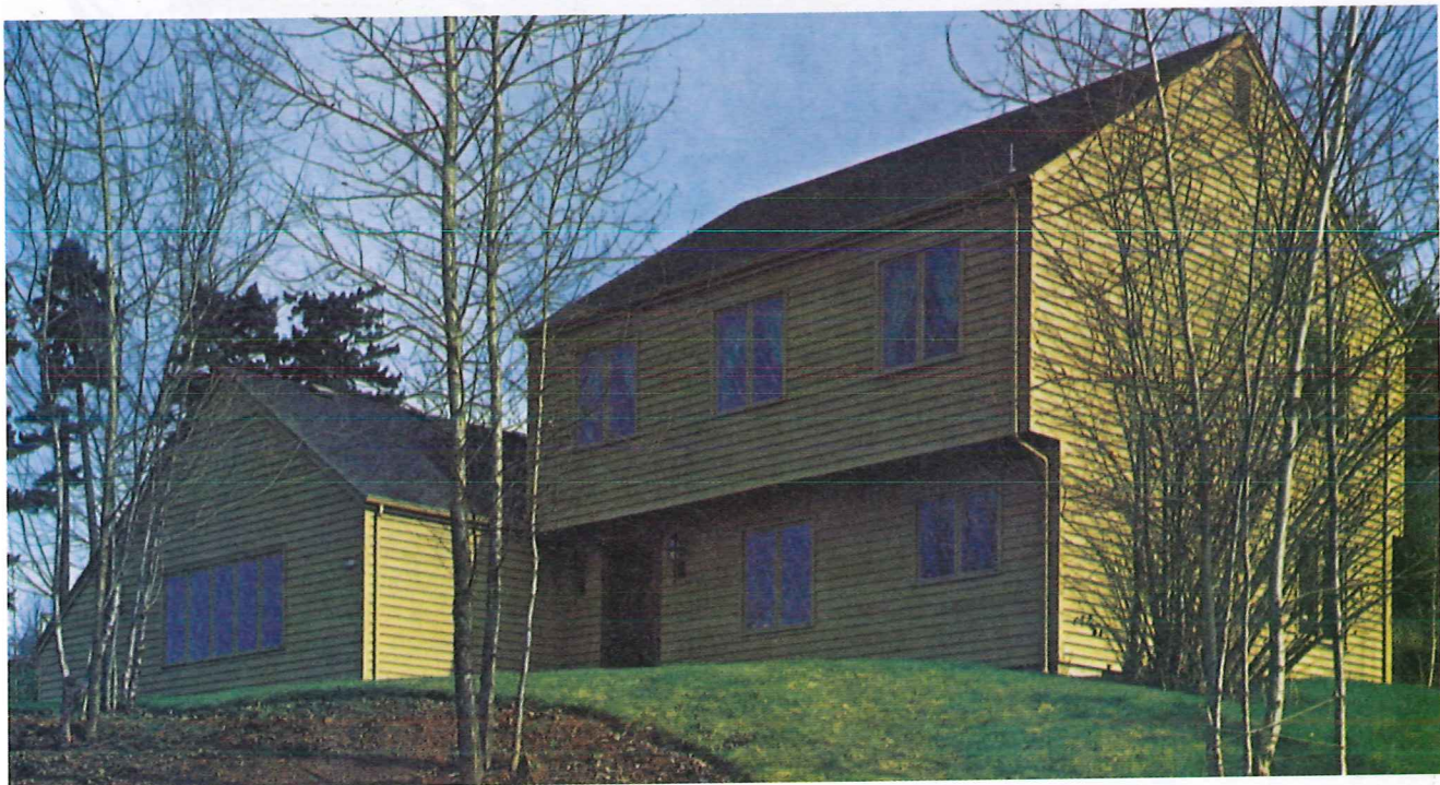
Figure 1-7. A contemporary Garrison home retains the straight-line features and overhanging second story of the original style.
