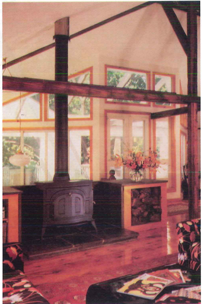
Figure 17-23. A wood-burning stove suitable as a local heating source for this large family room. Heat radiates from all sides of the stove. (Vermont Castings)
