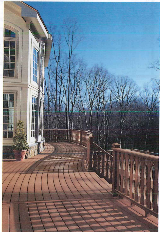
Figure 8-62. This multilevel deck enhances the architectural design of this home. (Trex Co.)
