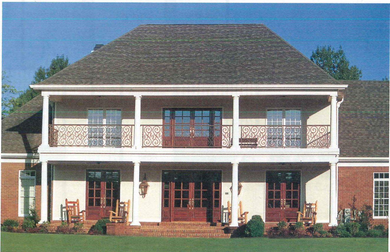
Figure 8-31. This main entry is clearly defined and centrally located to ensure easy access to the different areas of the house. (Photo Courtesy of James Hardie® Siding Products)
