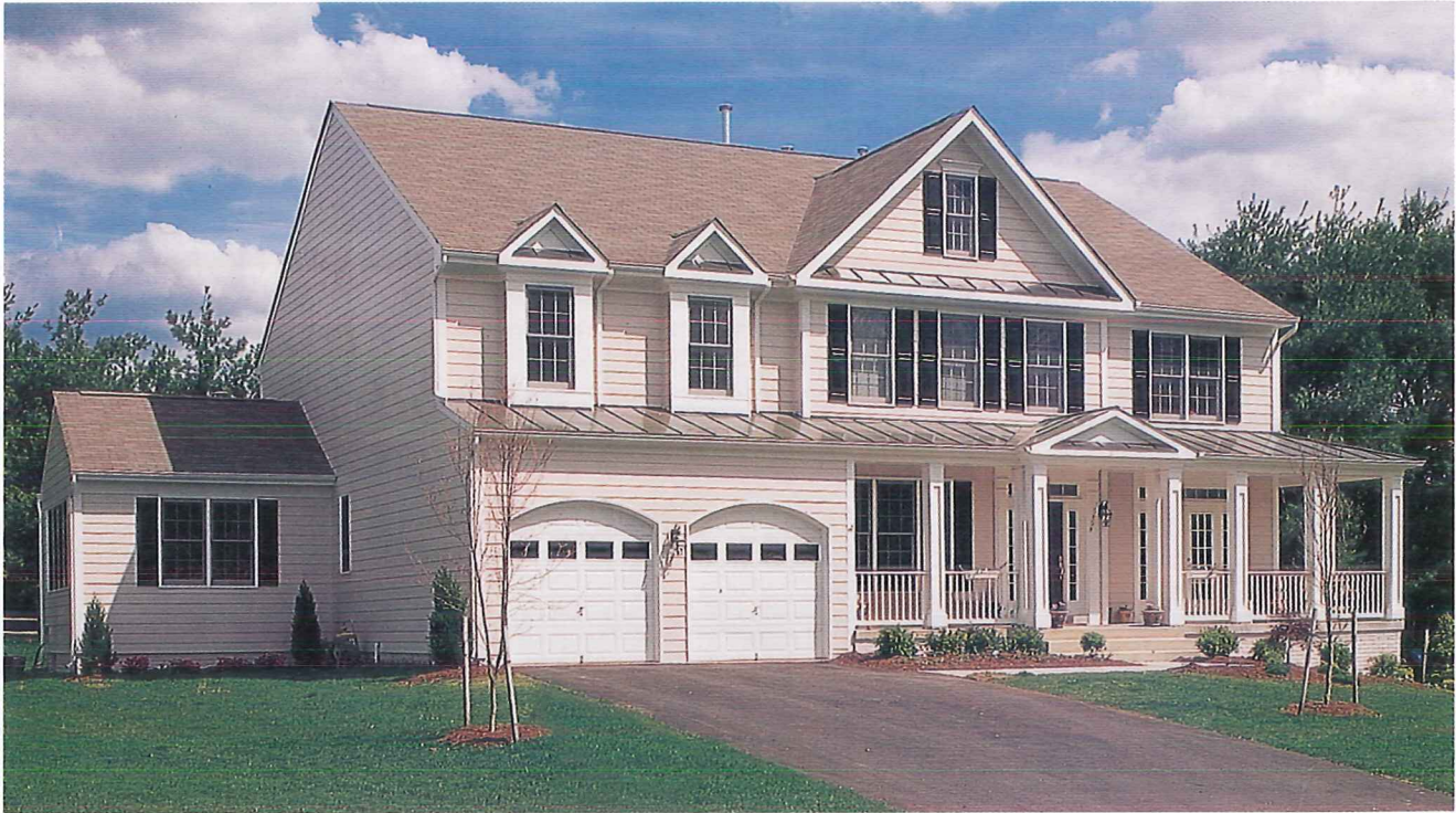
Figure 8-65. This front porch is an integral part of the house. It does not appear “tacked-on” to the house. (Photo Courtesy of James Hardie® Siding Products)
