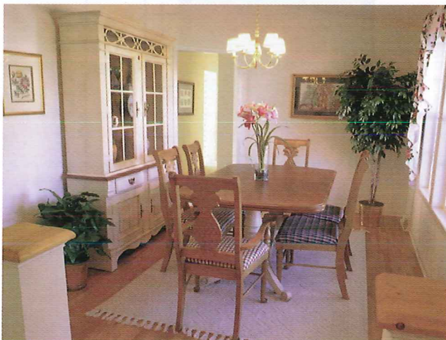
Figure 8-18. A dwarf wall separates the dining room and living area in this open plan. (Manufactured Housing Institute)
