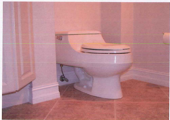
Figure 7-27. A contemporary one-piece water closet.
