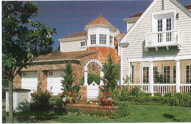
Figure 9-37. The two-car garage on this house is well designed to be an integral part of the style of the house. (Photo Courtesy of James Hardie® Siding Products)
