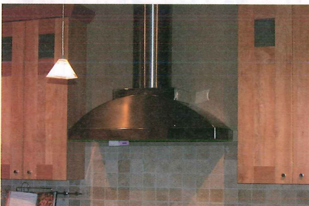
Figure 9-23. This unique range hood has charcoal filters to reduce odor. It is large and efficient in removing odors.
