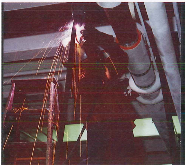
Figure 26-3. In gas metal arc welding (GMAW), a metal filler wire is automatically fed into the weld area. (Lincoln Electric)
